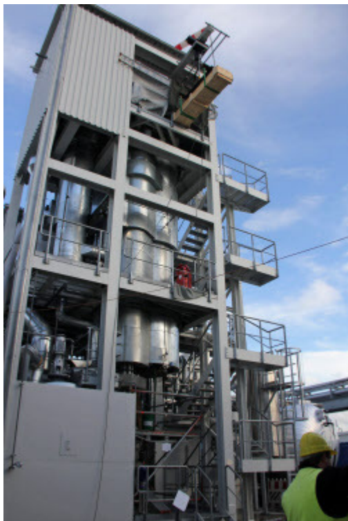
Figure 2: Audi's "e-gas" plant
