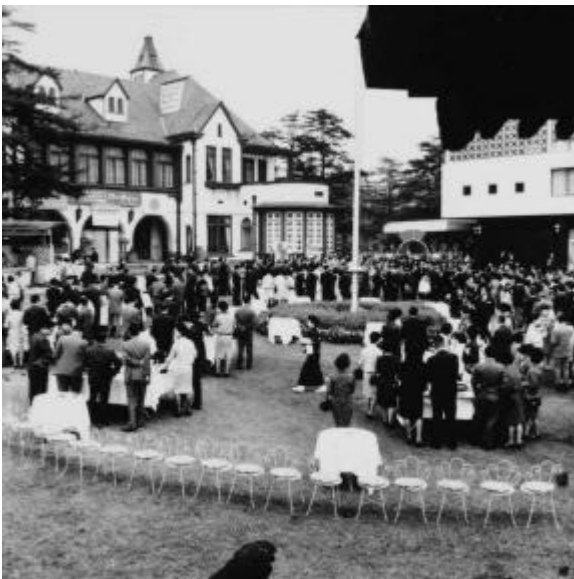
A scene of a garden party held in former Akasaka-prince Hotel. Photographed in 1965. Figure 15
